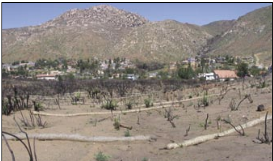
Figure 30—Fiber rolls do not reduce erosion but trap sediment on the slope. Where high values are at risk identify the emergency objective and select the treatment which best meets that objective.
