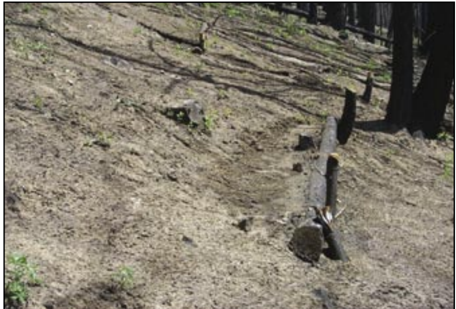
Figure 27—Once the LEB fills, sediment will move over or around the log. Soil berms on the sides of LEBs help hold more material behind the log.
