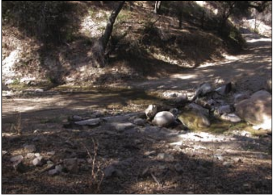
Figure 77—Ensure adequate length of the endwall and armor the outlet to prevent scouring.
