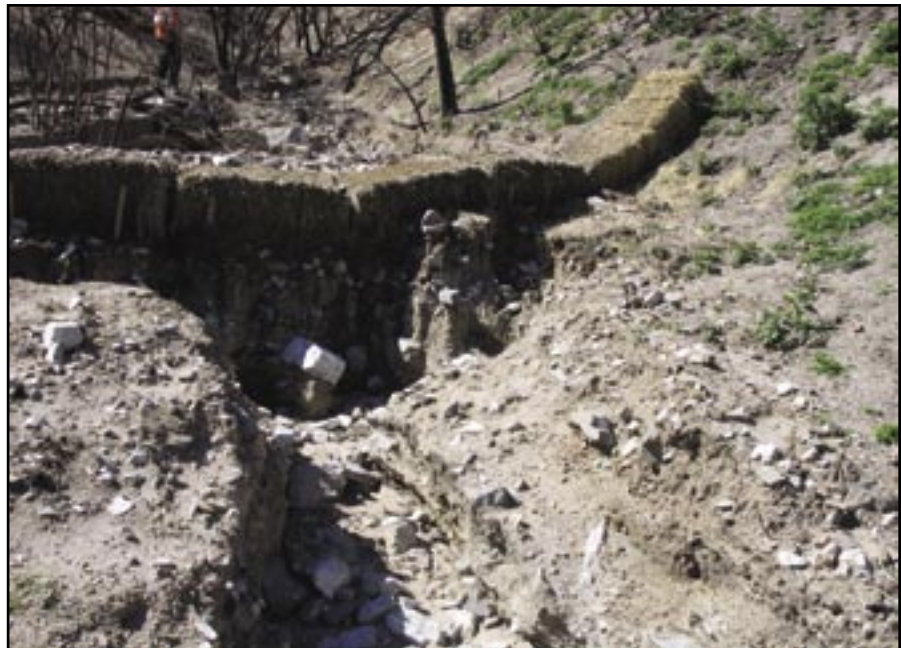
Figure 49—Strawbale checkdam that filled, overtopped, and created a gully below the structure.
