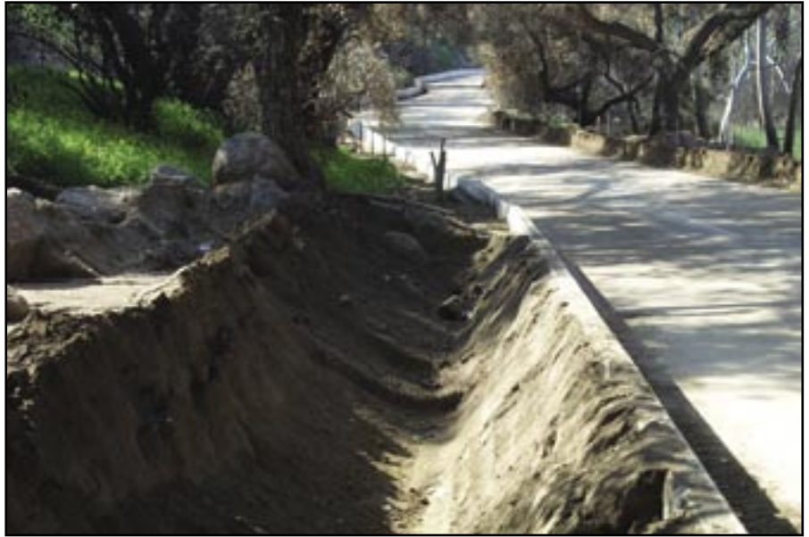
Figure 103—Jersey barriers (k-rails) line this road to protect vehicles on the road from debris flows.
