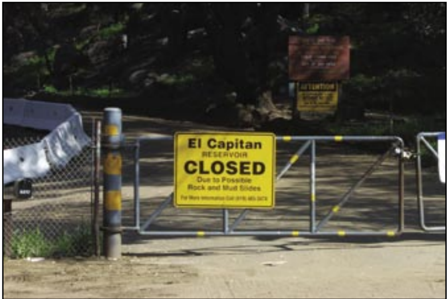
Figure 104—Gates prevent access to hazardous areas.
