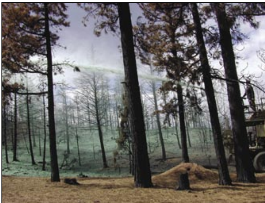
Figure 6—Ground application of hydromulch.
