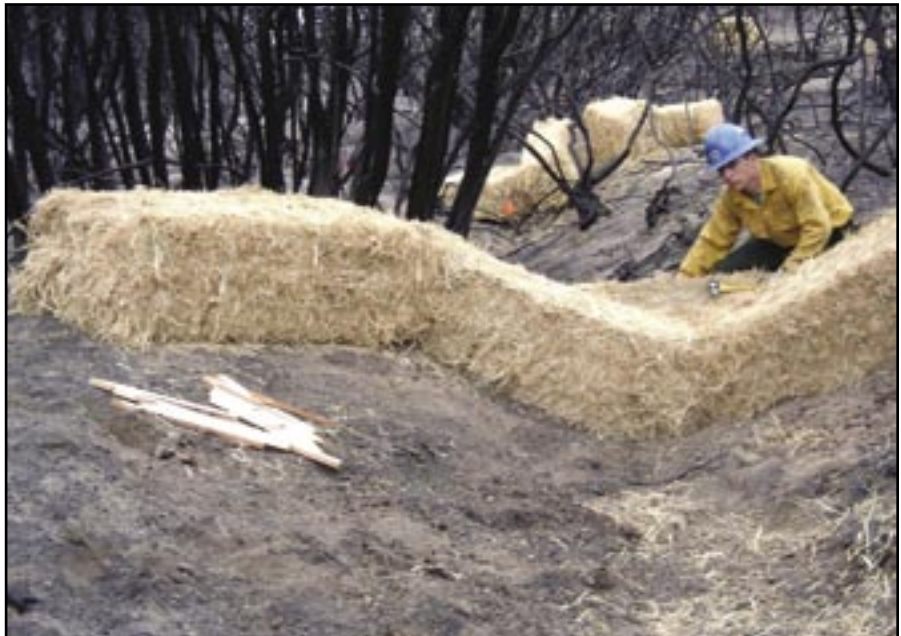
Figure 55—Install checkdams to avoid endruns.
