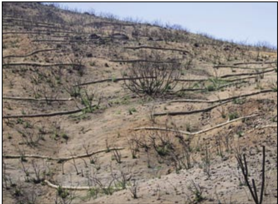
Figure 28—Fiber roll placed across the hillslope. Not all the fiber rolls are on the contour which can accelerate erosion.
