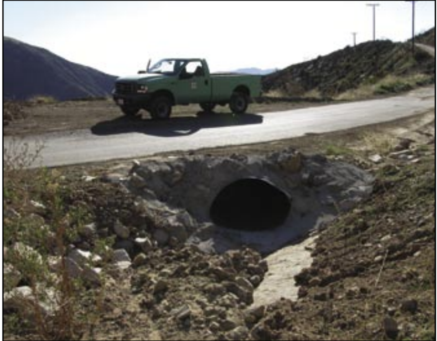
Figure 79—This larger pipe was installed to replace an undersized culvert that had failed in the past.
