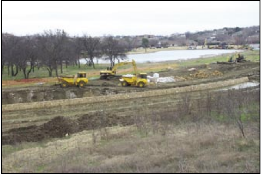
Figure 94—Typical equipment used to cleanout basins include excavators, backhoes, and dumptrucks.
