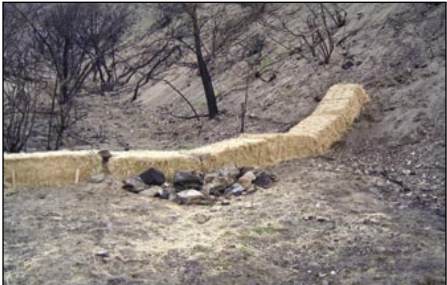
Figure 48—Strawbale checkdam with energy dissipater.
