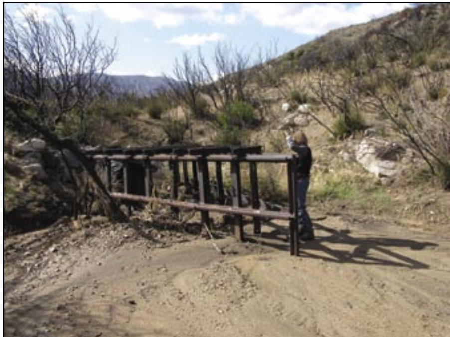
Figure 85—Debris deflector is located at inlet of culvert..
