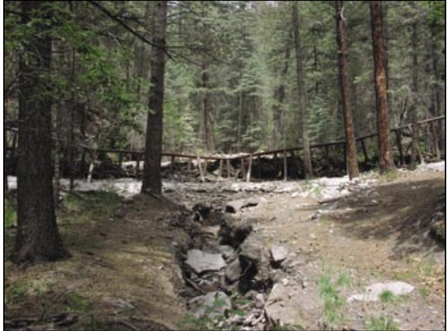
Figure 84—Debris racks must be long enough to avoid material from outflanking the structure.
