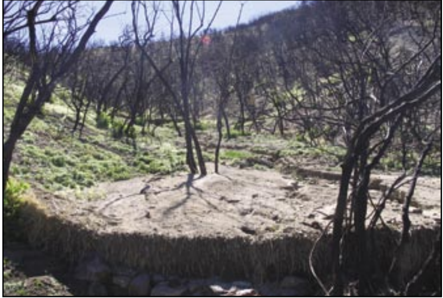
Figure 54—Checkdams should be inspected and maintained.
