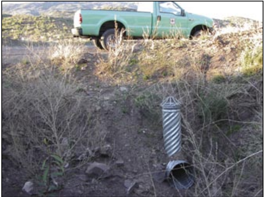
Figure 90—Riser is attached to prevent plugging of culvert.
