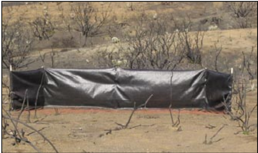
Figure 33—A recently installed silt fence.
