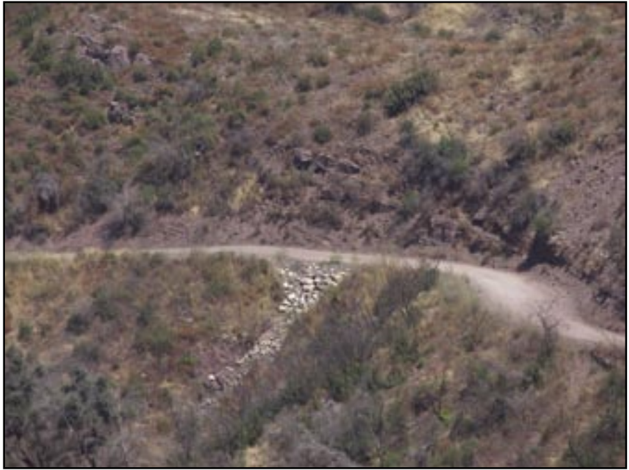
Figure 72—Rock armor used to replace failed overside drain.
