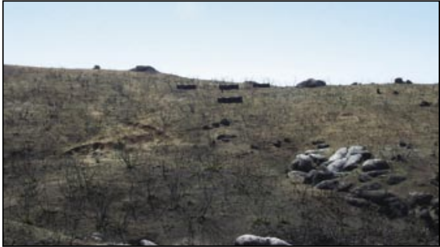
Figure 35—Silt fences are effective at trapping sediment but require inspection and maintenance. Silt fences should be removed once the area has stabilized.
