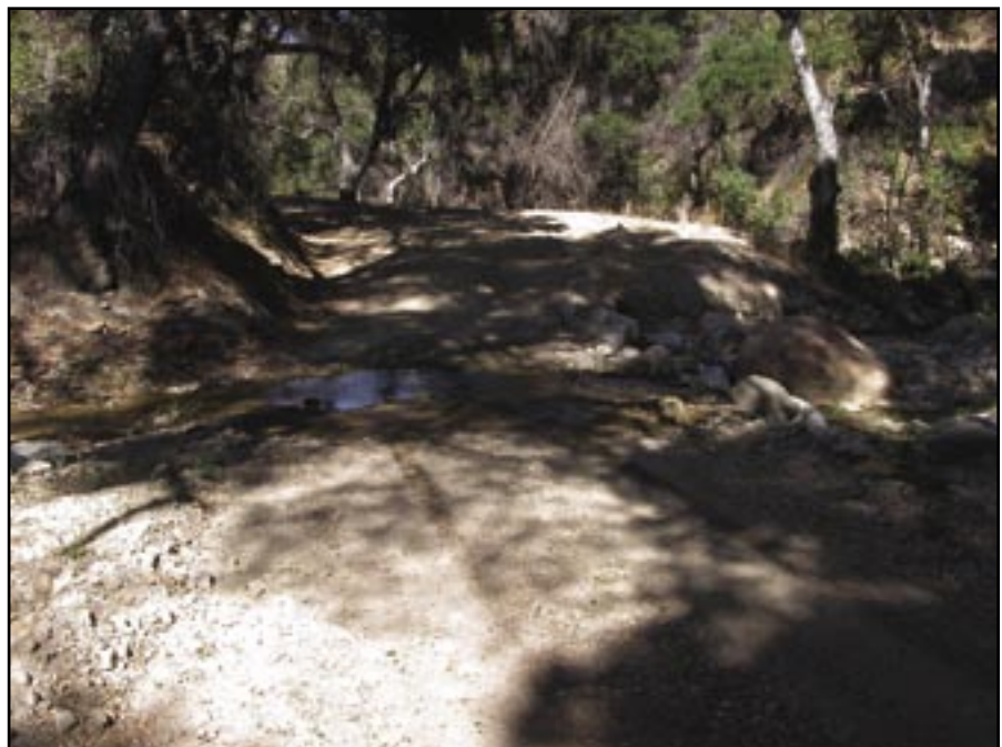
Figure 76—Low-water stream crossing replaces a 24-inch culvert.
